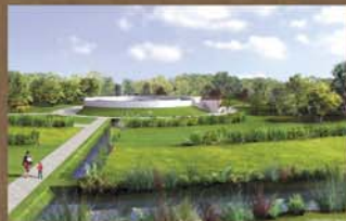
Eco-construction HQE® of the sewage treatment plant of Buis-la-Riv. - France - 2007
