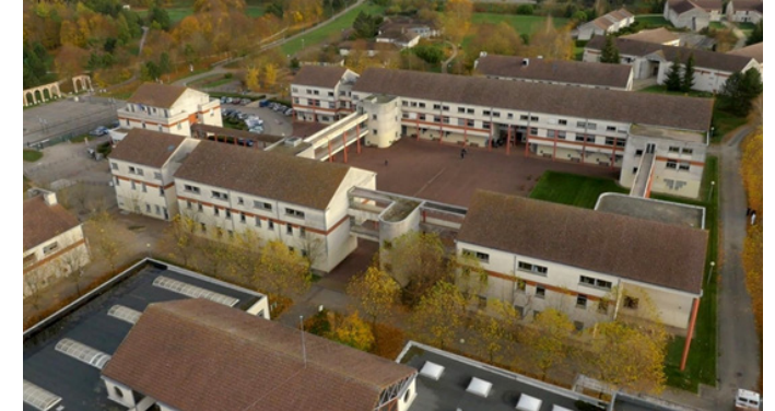
View of Edouard Herriot High School in SAINTE-SAVINE (10), FRANCE
