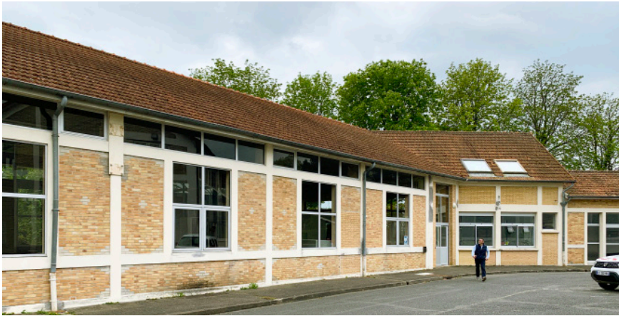
Main building Longueville Factory - Longueville (77), France
