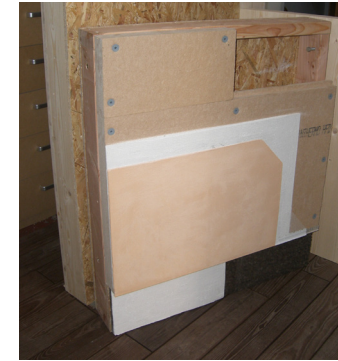
Constructed walls with natural thermal insulation
