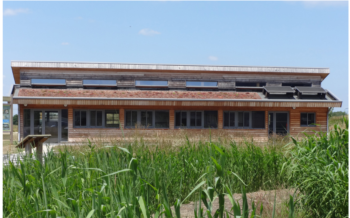
View on the bioclimatical operating building
