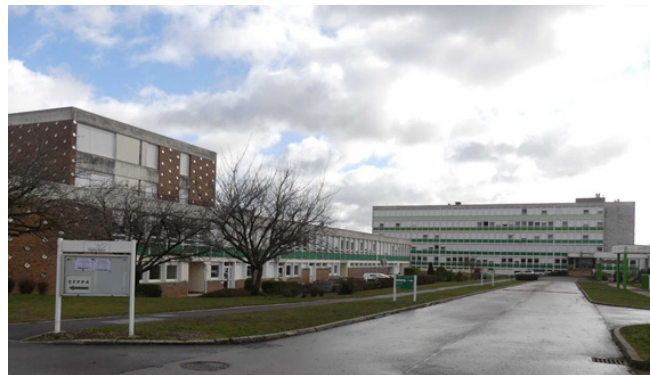
View of EPLEPPA SAINT-POUANGE SITE (10), FRANCE
