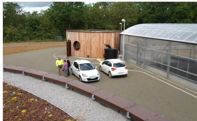
View from the operating building, june 2012
