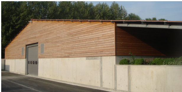
View on the terminated project
