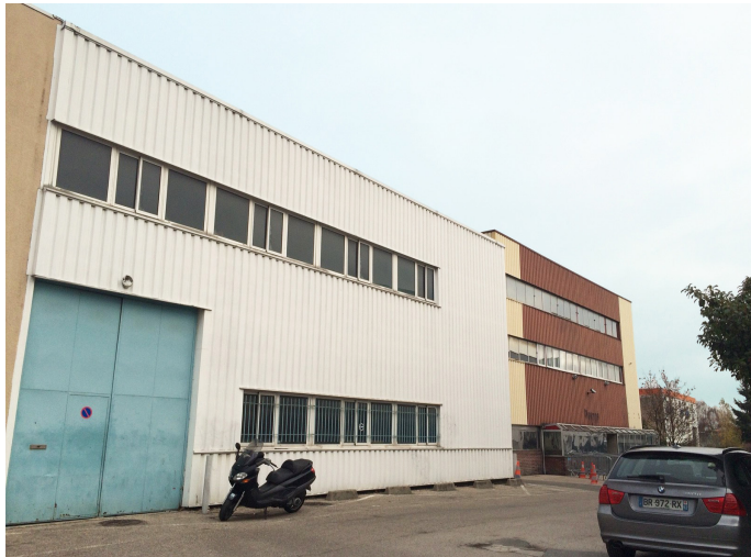
View on the existing building "CYPREOS"
