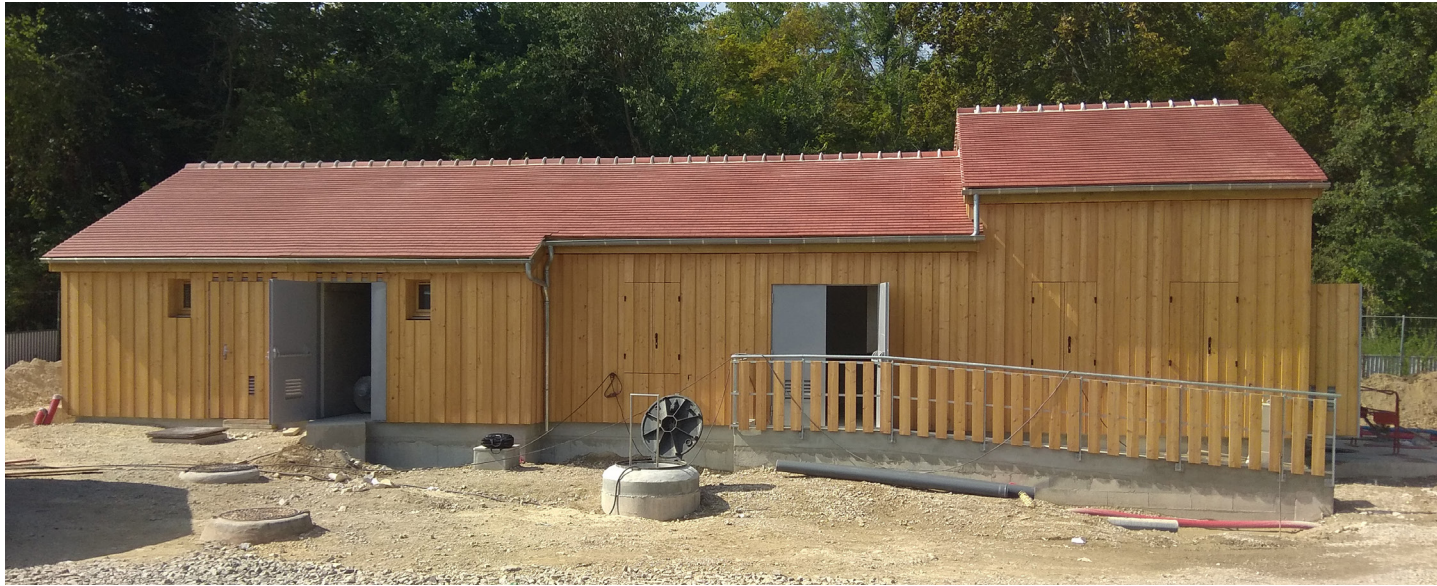
Photograph of the lifting station - South West view
