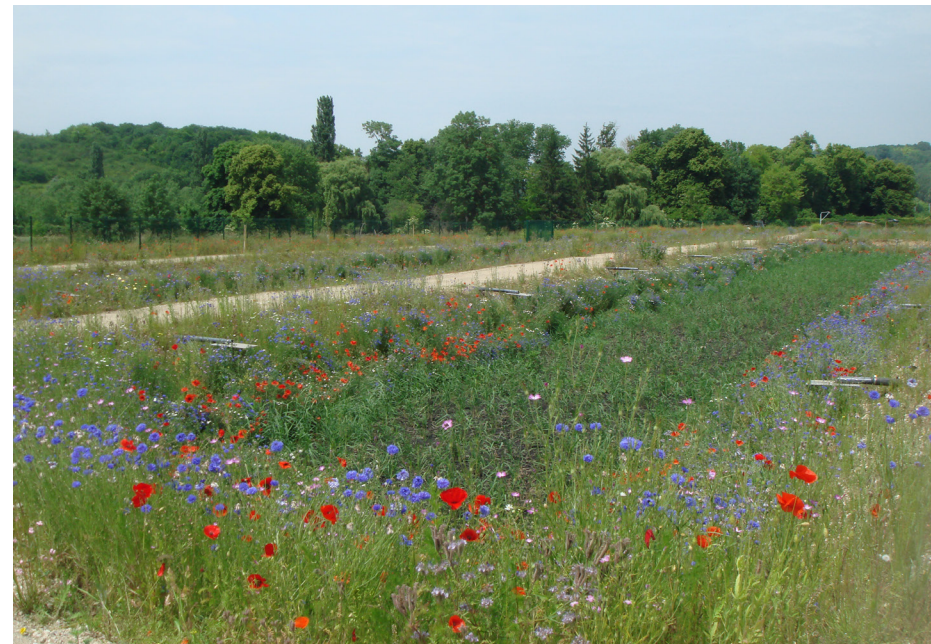
Reed beds (4 000 m 2 ) to treat sewage water
