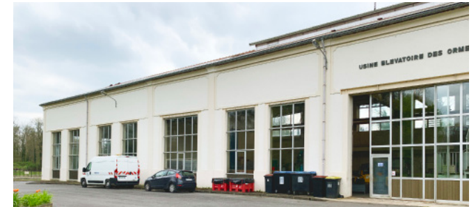
East Facade Ormes Factory - Les Ormes-sur-Voulzie (77), France
