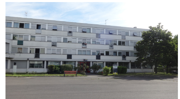
View of Paul Eluard's high school in SAINT-DENIS
