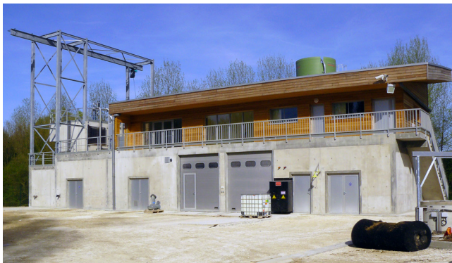
View on the operating and technical buildings
