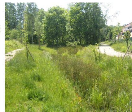
Example of a planted ditch.
