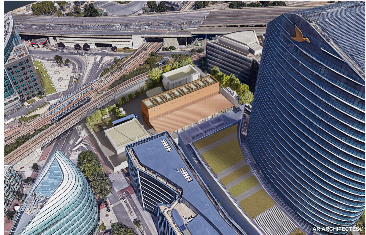
View of the building in the urban and dense site.
