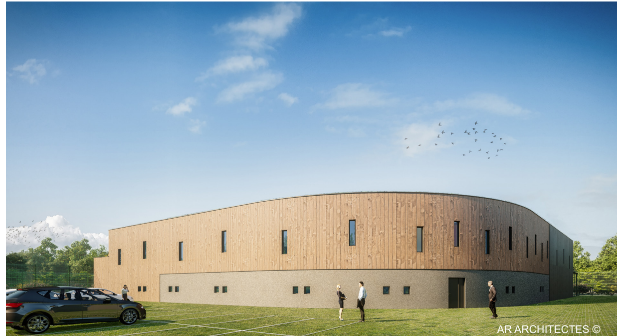
View of the entrance on the south side, bioclimatic technical building in pre-grayed larch wood cladding, textured concrete and metal cladding
