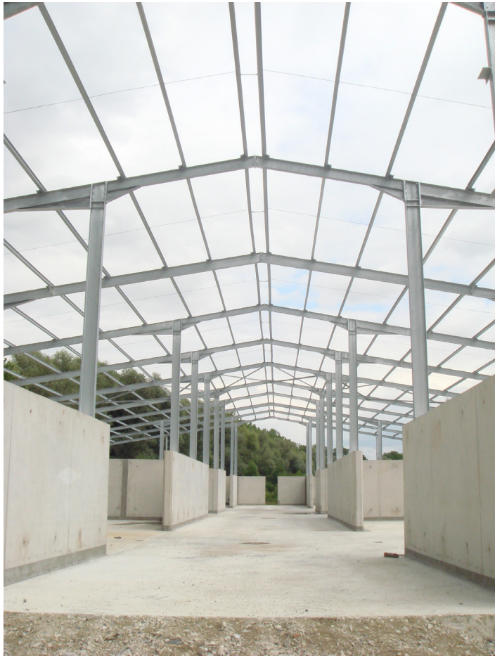
View on the structure of the construction
