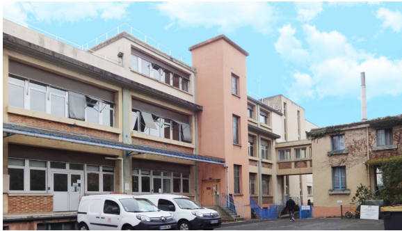
Current facade of Building C
