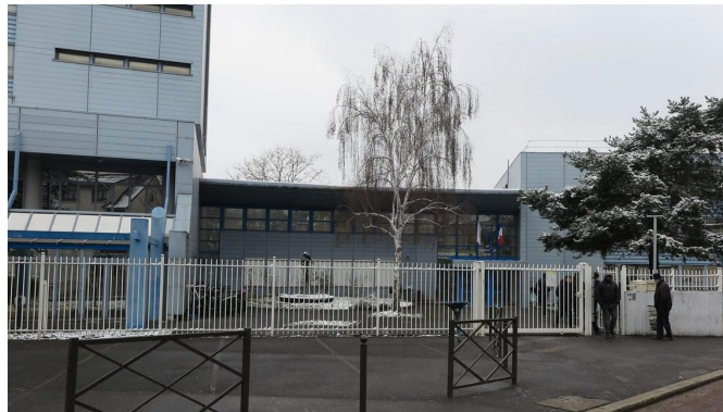
A view of the Jean Jaurès' high school in ARGENTEUIL
