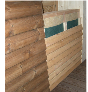
Constructed walls with natural thermal insulation
