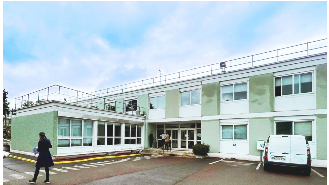
Main facade of the C1C2 building of the Vésinet site of the IRSN
