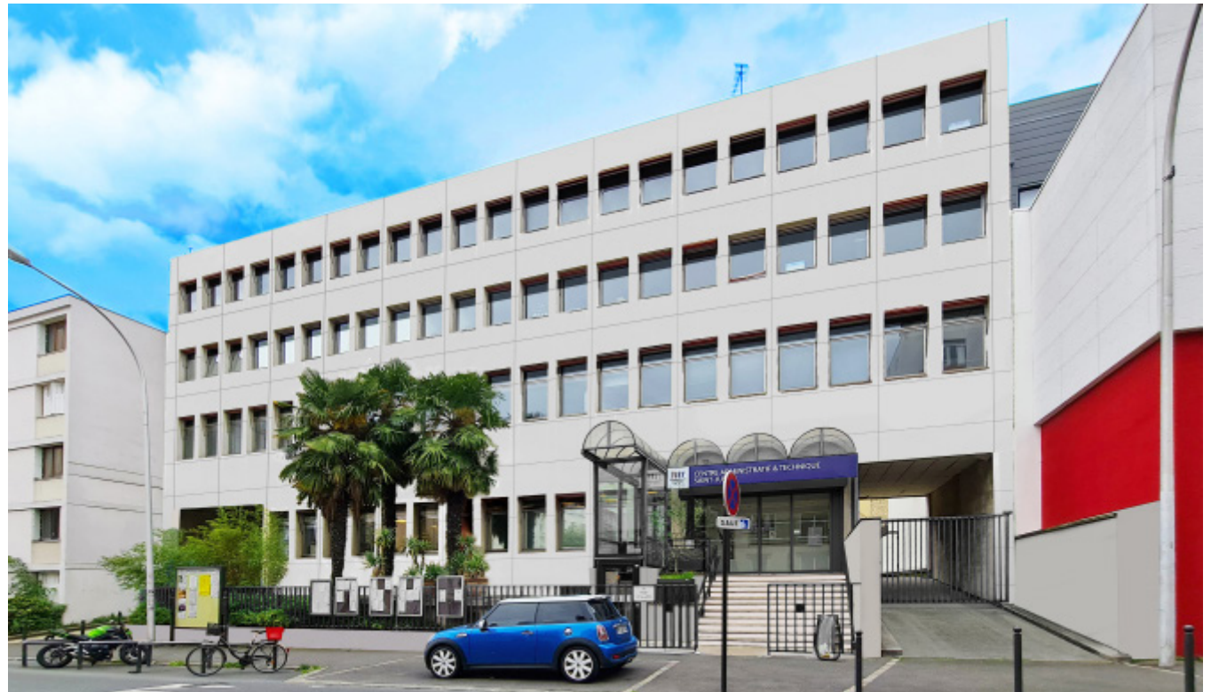
Main entrance facade of the Saint-Just Administrative Center after the energy-efficient renovation
