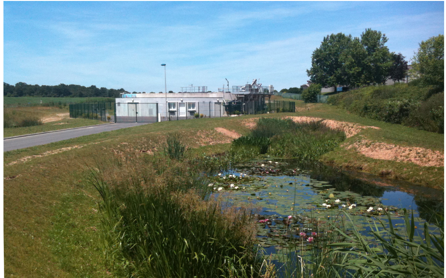
View on the entrance of the plant. Two constructed wetlands are designed outside of the road
