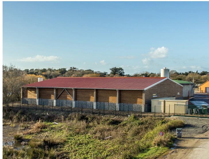
View of the industrial building for mud
