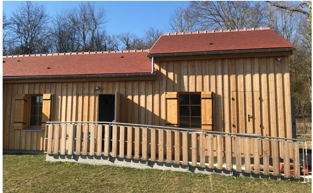
Photograph of the lifting station entrance
