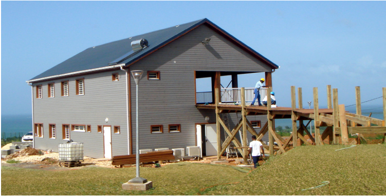
View of the house of environment
