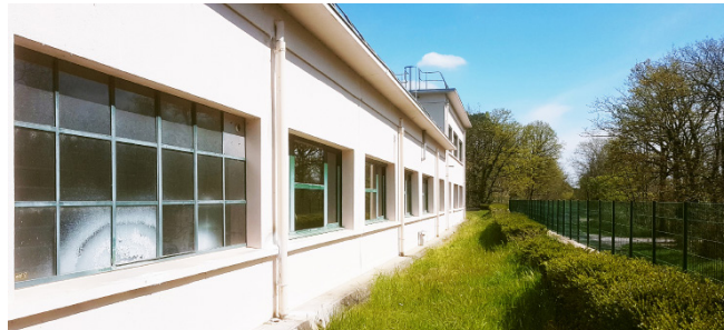
Building A Sorques Factory - Montigny-sur-Loing (77), France
