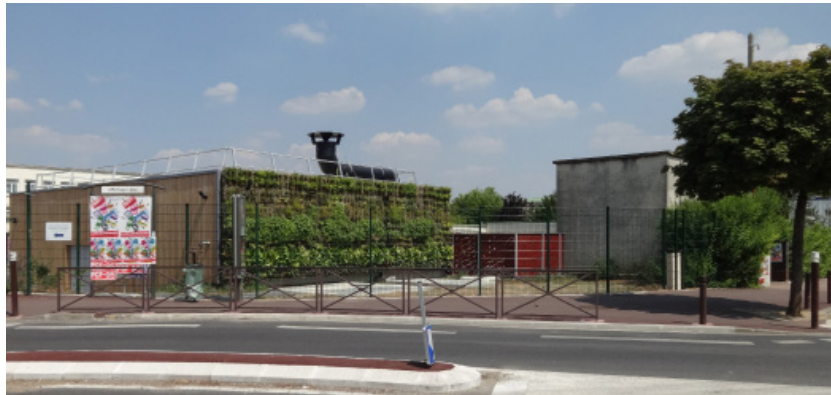
View from Louis Savoie street
