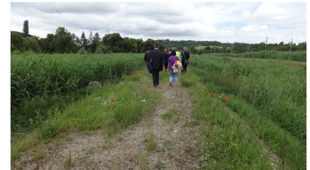
Visit of the reed bed for sludge depolution coming out of the plant.
