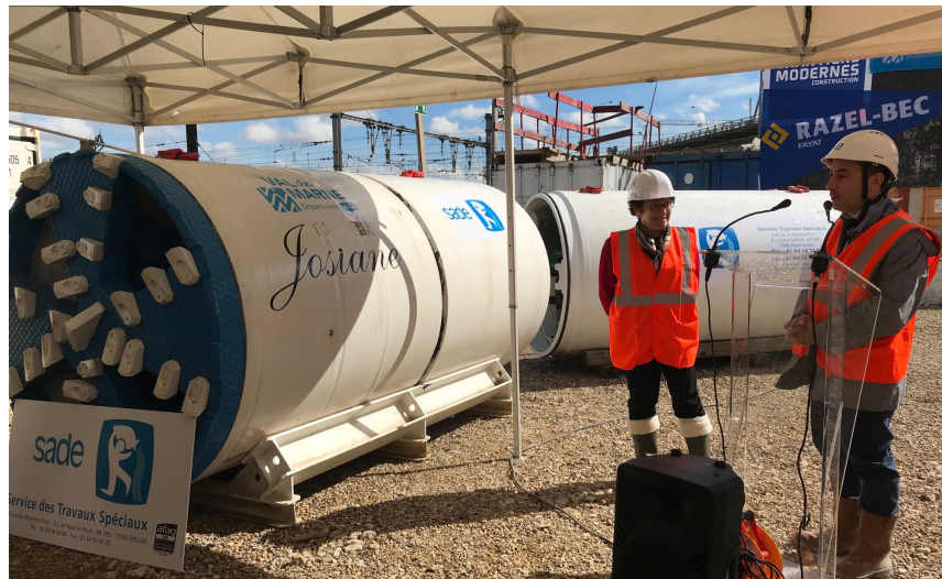
Baptism of the microtunneling "Josiane"
