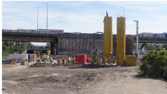
Construction site, entrance of Vitry-sur-Seine
