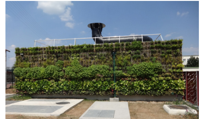
View from Est street on the green wall on the South
