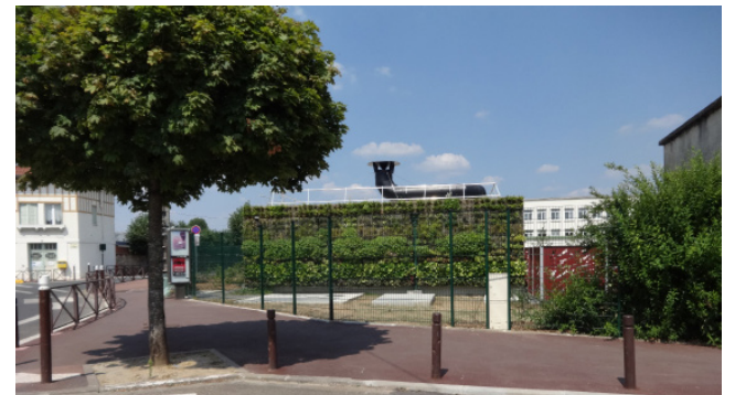
View from East street
