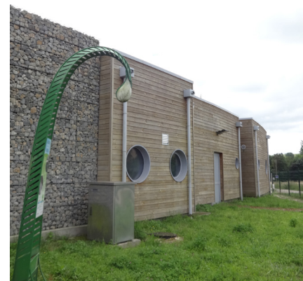
Bioclimatic wooden operating building.
