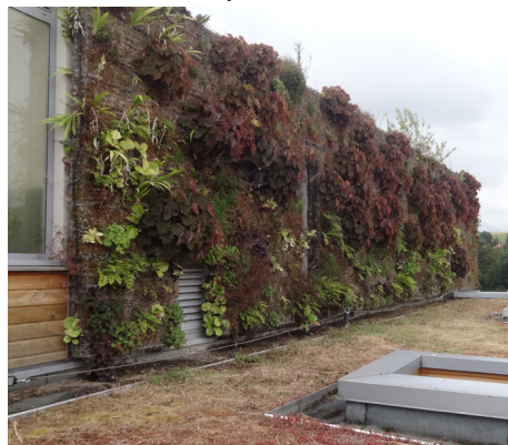
View on the green wall and roof.
