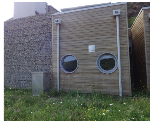
Bioclimatic wooden operating building.
