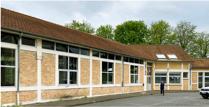
Main building Longueville Factory - Longueville (77), France
