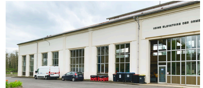
East Facade Ormes Factory - Les Ormes-sur-Voulzie (77), France
