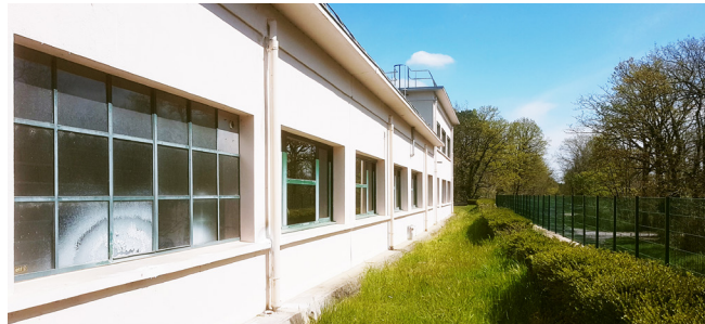
Building A Sorques Factory - Montigny-sur-Loing (77), France
