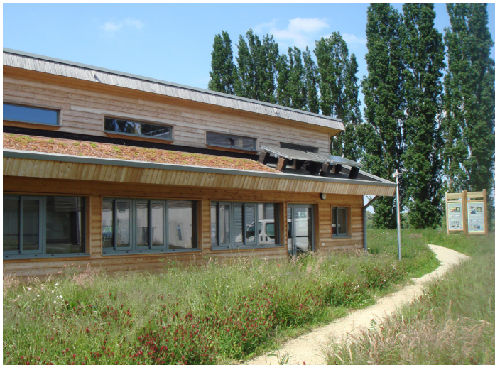
View on the operating building
