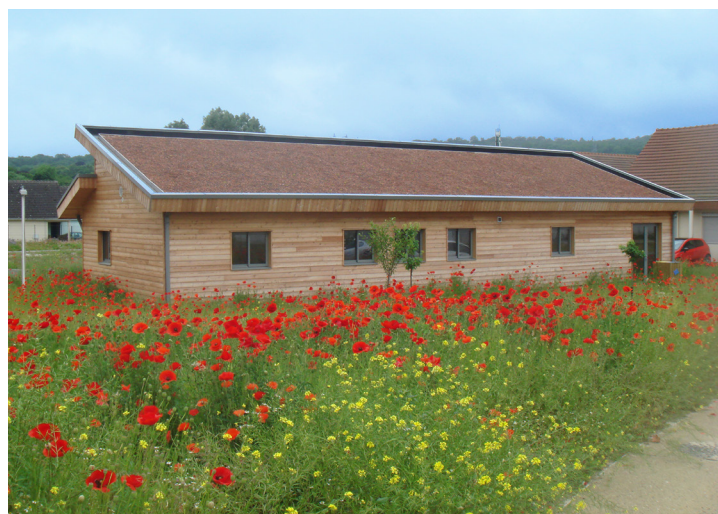
View on the reconstructed landscaping surrounding the building
