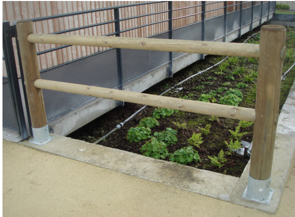
View of the air treatment filter with a surface of 28m 2
