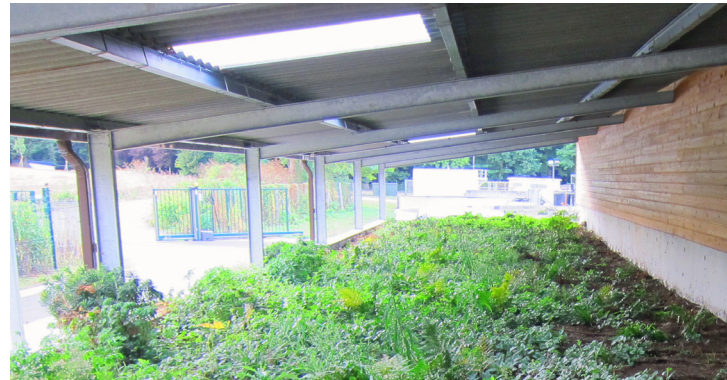
Treatment of 72 000 m 3 /hour on an area of 135 m 2 of green planted filter
