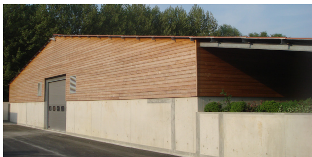
View on the terminated project
