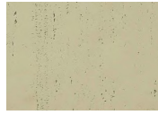
Precast concrete panel (smooth matrix)
