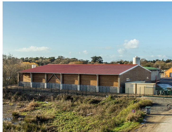
View of the industrial building for mud
