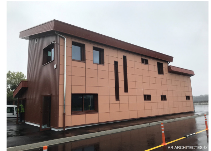
Photo of the south-west facade in terracotta and aluminium
