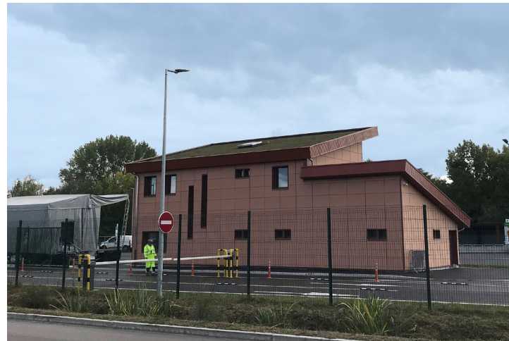
Photo of the environmental recycling waste plant
