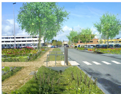
Water coming out of the channel is collected through filtering green ditches. These ditches direct water to the river "La Bourbince".
