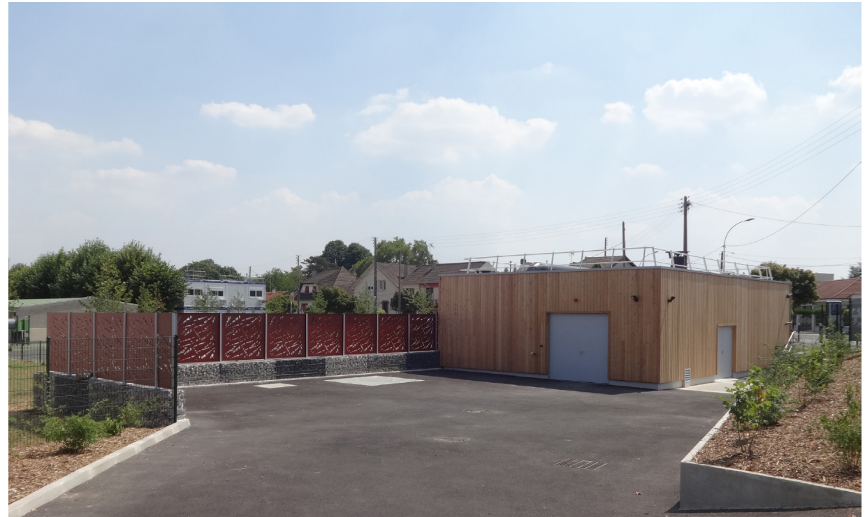
View of the entrance, gabion cladding associated with the metal fence, eco-plant in wood
