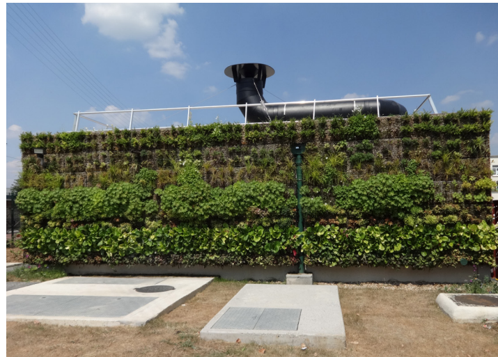
View from Est street on the green wall on the South
