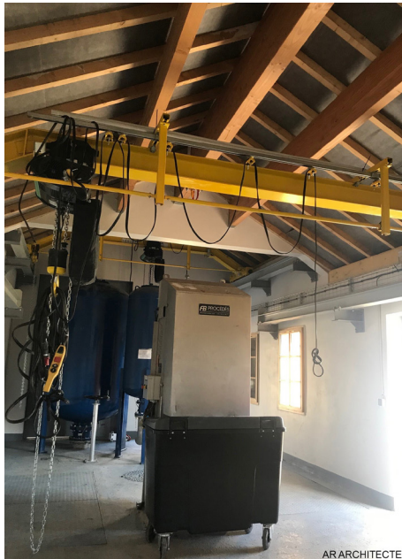
Wood frame structure
