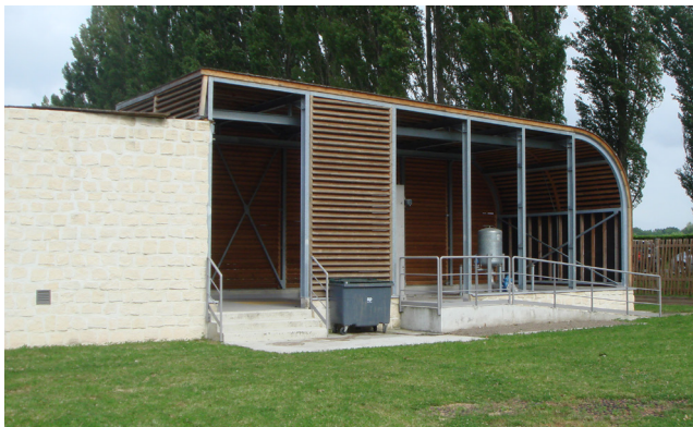
View on the technical post PR7
