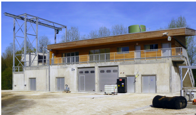
View on the operating and technical buildings
