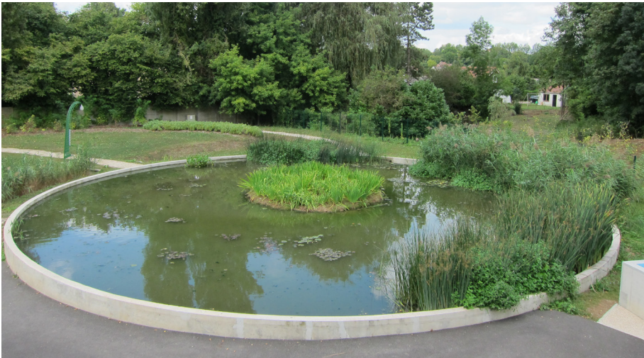
View on the recycled civil work into and an aquatic garden
