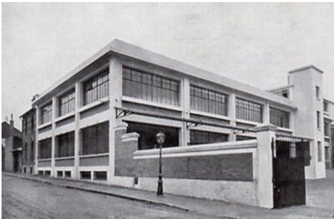
Building C of the Saint-Just Administrative Center - The former Lesquendieu perfume factory built in 1930
