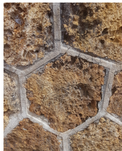
Millstone support joints restored to original condition
