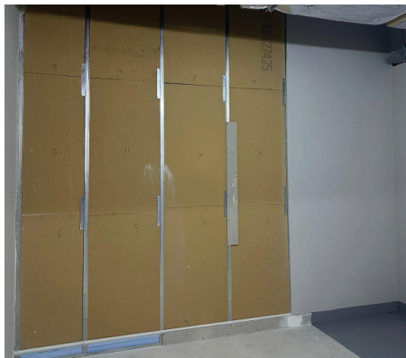
Internal insulation with wood fiber
