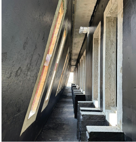
Interior of the wall before earth infill
