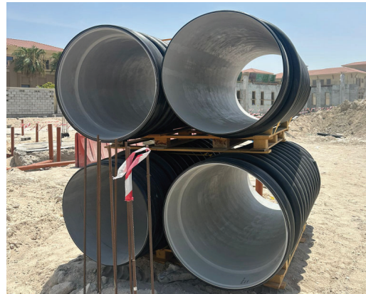
Canadian well duct with a diameter of 800 mm
