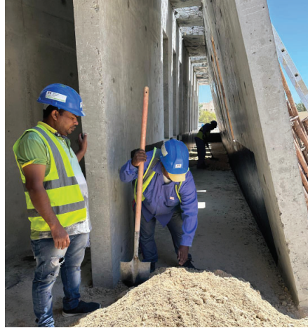
Earth infill of the south wall
