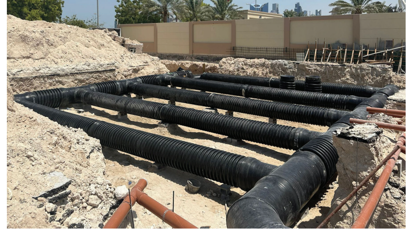
Installation of the Canadian well, residential side (AHU 8000 m 3 /h)
