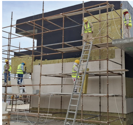
Rock wool insulation beneath stone cladding
