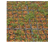
Vegetated cellular paving
