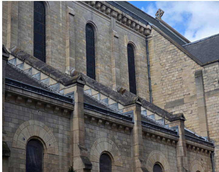
The zinc flashing on the parapet walls and the zinc gutter.
