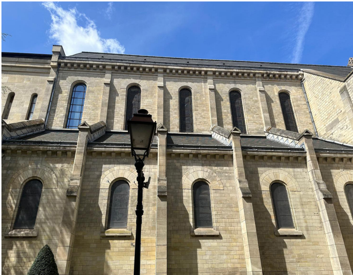
The replacing the slate roofing.
