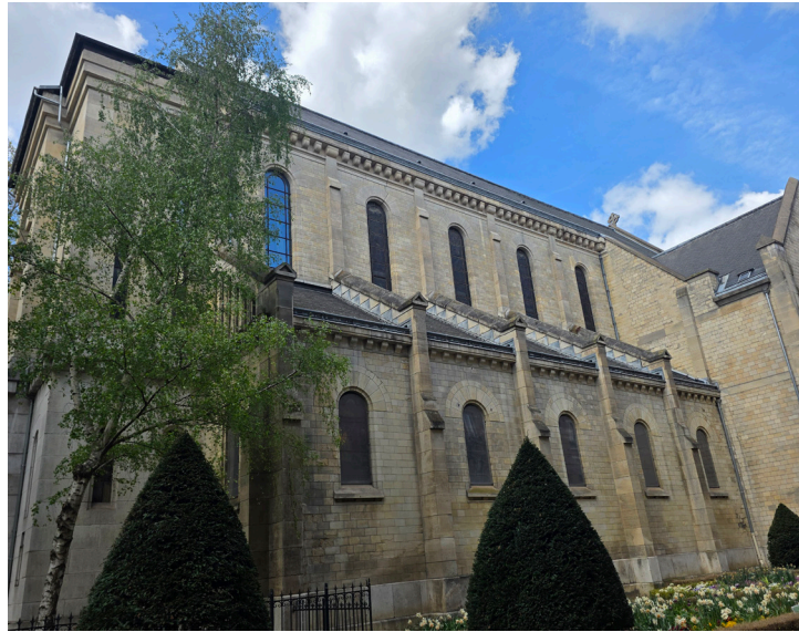
The lean-to roof covering the side aisle of the Saint Vincent de Paul church, located to the southeast of the building.
