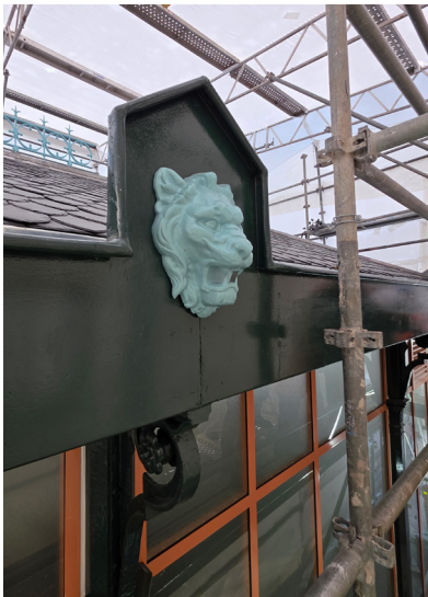
Metal framework restored to its original condition - RAL 6012 color Joinery replaced with new ones - RAL 3012 color Lion head antefixes restored to their original condition - RAL 6034 color
