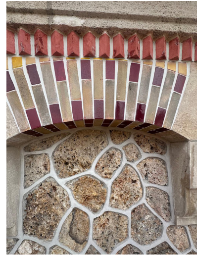
Lime plaster joints in an off-white shade of gray for the restored retaining walls, laid in a straight, geometric pattern along the contours of the rubble stones. Joints for the exterior tiling (glazed bricks, brick frieze) are finished with lime plaster in RAL 1013 (pearl white).
