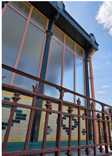
Metal framework restored to its original condition - RAL 6012 color Joinery replaced with new ones - RAL 3012 color Lion head antefixes restored to their original condition - RAL 6034 color
