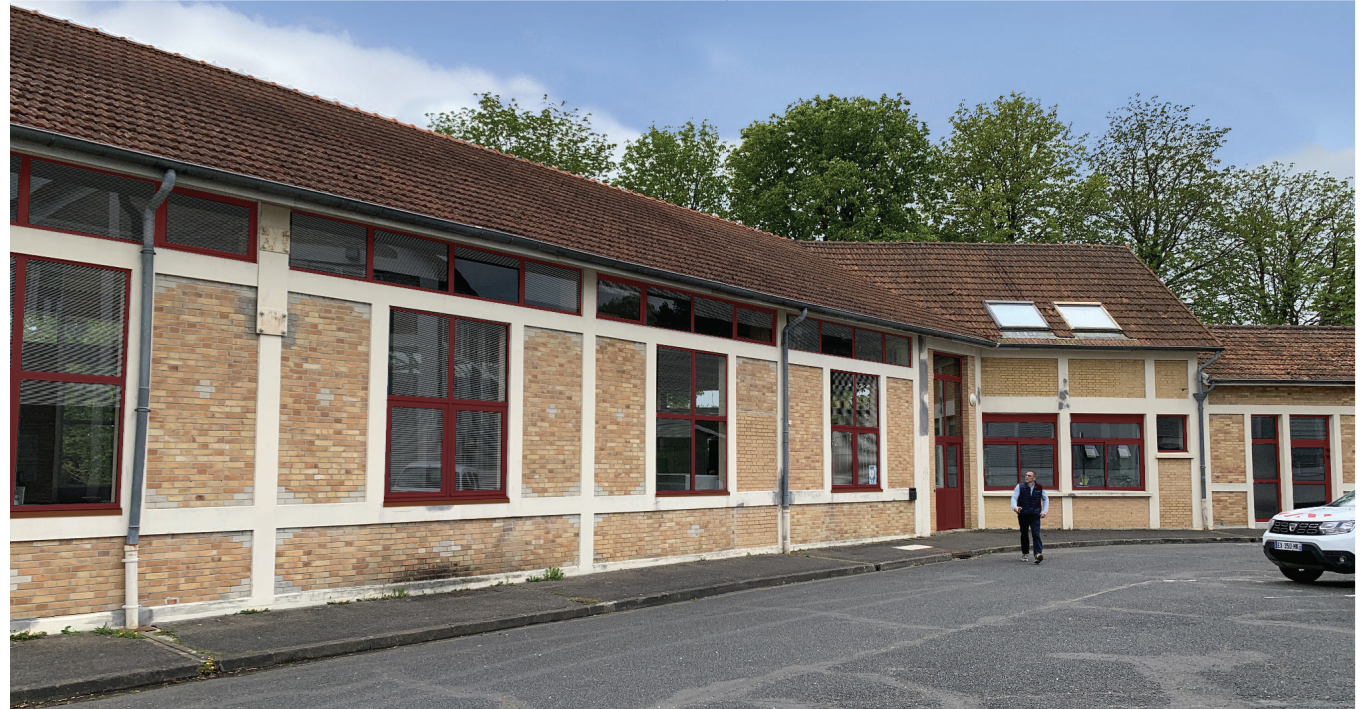
View of the north façades of the main operations building – projected state, restored in accordance with the original
