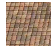
Aged roof tiles
